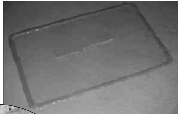
Patch with edge sealer applied.
