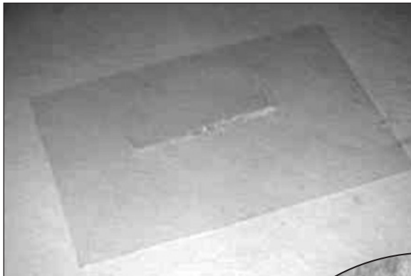
Clear film applied to roof.
